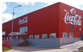
Coca Cola Plant Project (South America)
